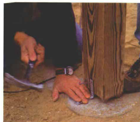
If uplift is unlikely, cheaper hardware anchors the posts. A cast-aluminum base keeps the post off the ground.
