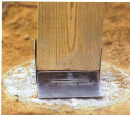
Anchor resists strong uplift. This anchor allows the post to be tweaked plumb before the nut is tightened.
